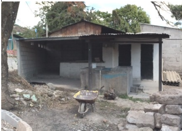
Crude feeding station near completion in Comoyagua, Honduras
